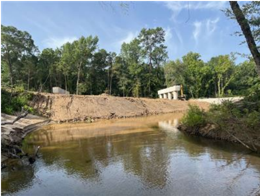
Figure 8. Roadway Construction on Stewarts Creek
