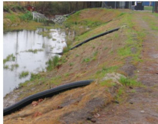
**Figure 15. Two examples of using slope drains for bank stabilization. Surface water generated during larger storms flowing into the wetland is directed into the drains. The drainage reduces erosion that would result from concentrated flow down the banks.**
