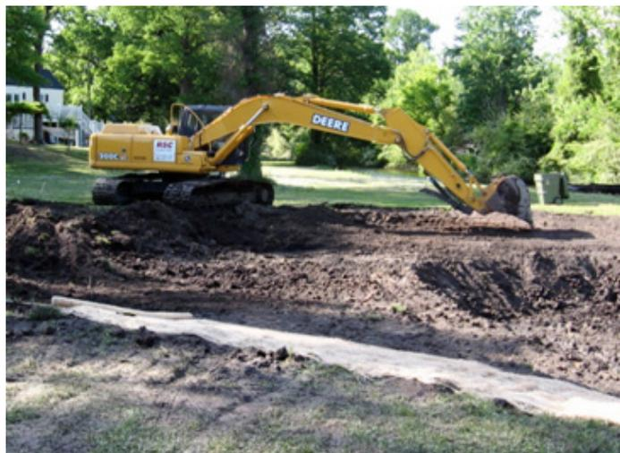
Figure 12. If possible, keep the excavator out of the wetland and use the bucket teeth for excavation to keep the wetland soil loose for planting. Remember to stockpile topsoil for replacement!
