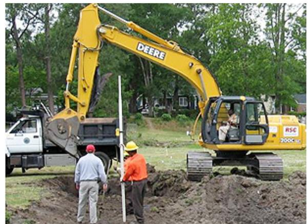
**Figure 11. Keep dump trucks moving for off-site transport of soil (top), and keep the excavator operator updated on correct grade to speed construction (bottom).**
