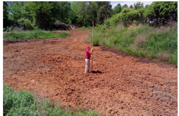
Figure 13. Surveying a properly prepared wetland surface.
