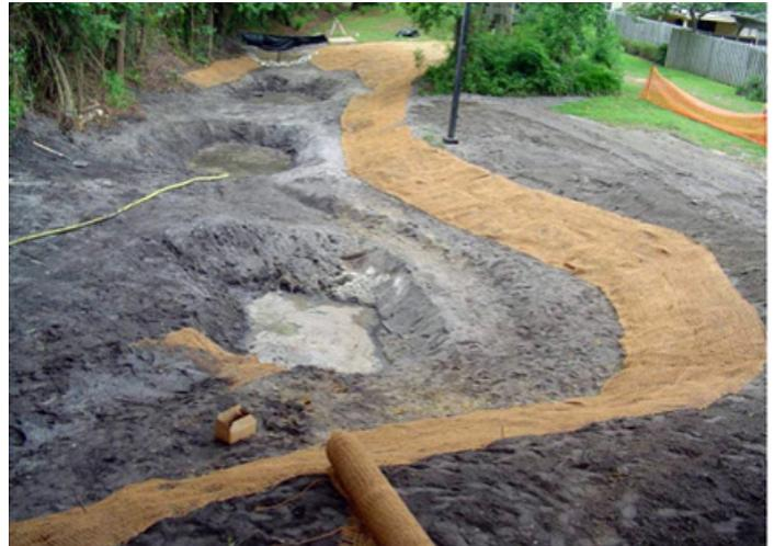
Figure 5. Stabilize the banks each day following excavation of a stormwater wetland.
