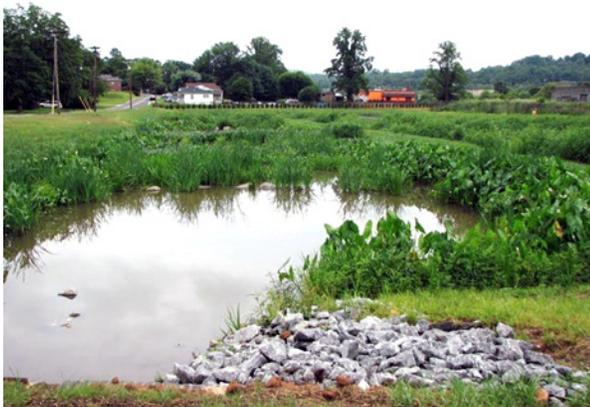
**Figure 19. Adding features and topsoil in a large wetland. Side-slopes have already been prepped, and grass is coming up (top). After 1 year, vegetation is successfully established (bottom).**
