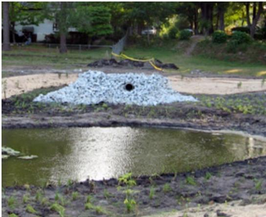
**Figure 16.** Use riprap of granite or marl to slow inflow to the wetland and protect the inlet from erosion.
