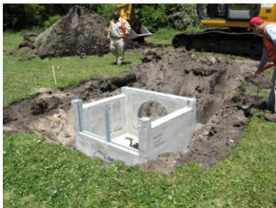
**Figure 8.** Examples of outlet structures built on-site (top) and prefabricated and delivered to the site (bottom)
