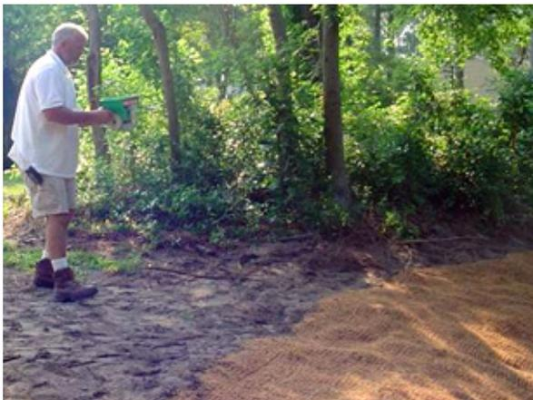
**Figure 14. Stabilize banks daily with lightweight fabric and seeding to reduce the chance of erosion while the wetland develops.**
