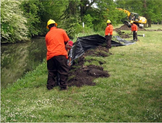
Figure 4. Installation of a silt fence along a stream bank near a new stormwater wetland construction site
