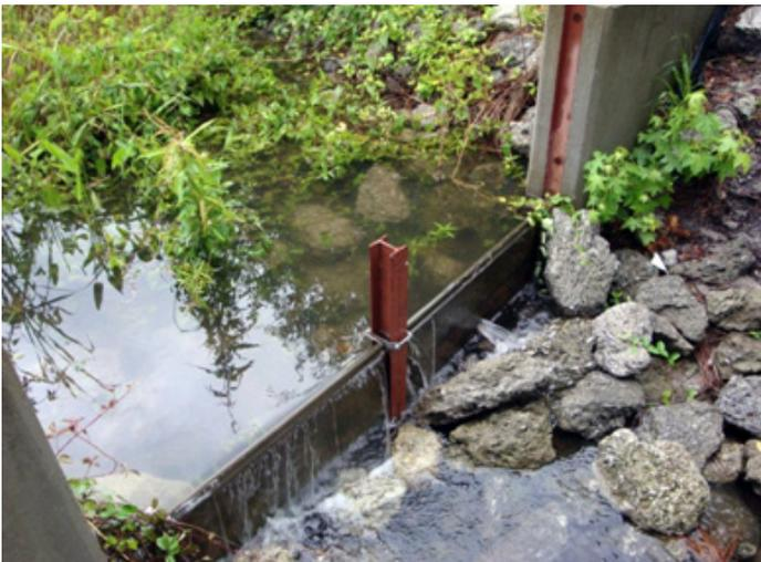
**Figure 10. Armoring downstream of the outlet structure will reduce the potential for erosion that could threaten stability.**
