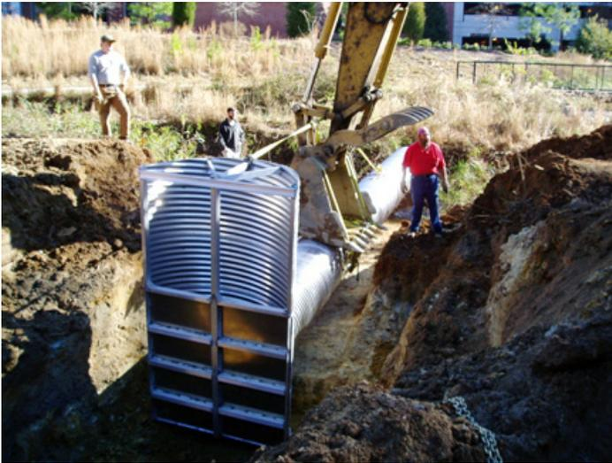
**Figure 9. Installation of a large flashboard riser outlet structure**
