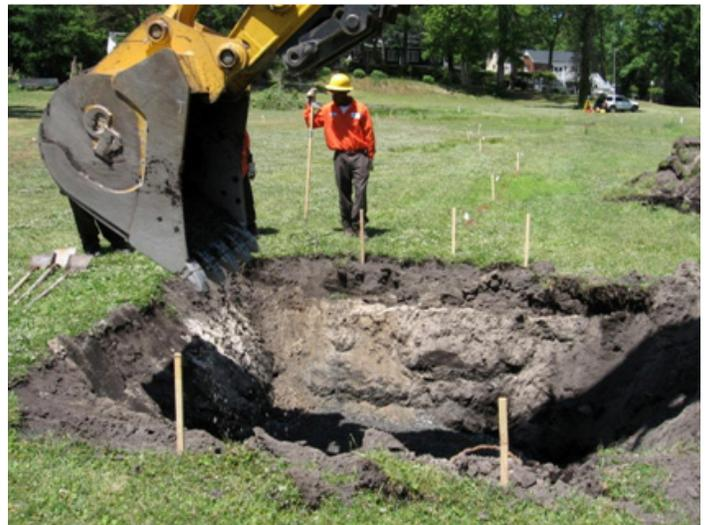
Figure 3. Stake out the wetland perimeter, internal wetland features, and locations of structures prior to excavation. Make sure all existing utilities at the site are located and marked.
