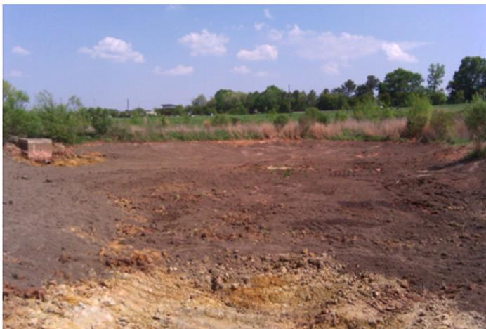
Figure 6. The soils for this stormwater wetland are properly prepared for water and wetland plants.
