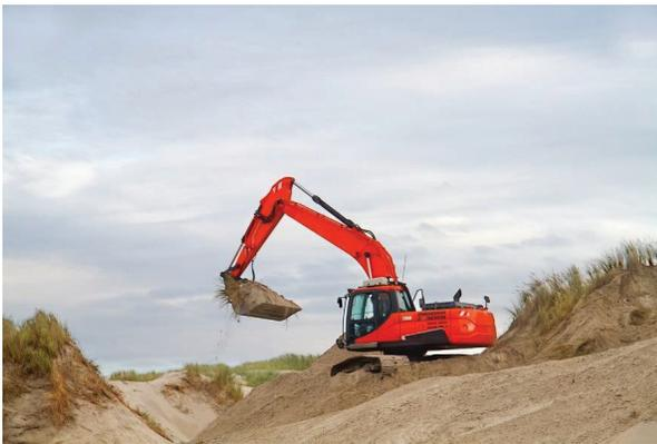
Beaches reduce the destructive impact from coastal storms by acting as a buffer along the coastal edge and absorbing and dissipating the energy of breaking waves. Beach nourishment and dune restoration are soft engineering alternatives to hard shoreline structures.
