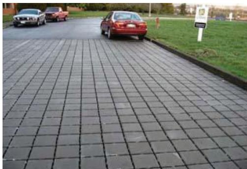
Permeable pavements have porous surfaces that slow, filter, and clean stormwater runoff.
