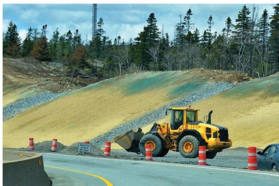
Vegetation cover is the most effective and practical means of preventing loss of sediment. The roots of vegetation bind soil particles together to resist erosion from runoff rainwater. Vegetation also absorbs the impact of raindrops to prevent the detachment of soil particles and reduces the velocity of runoff, which allows water to infiltrate.
