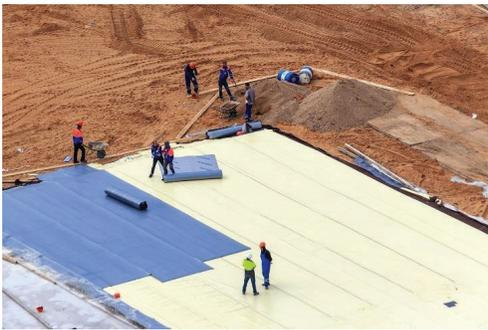
Geosynthetics/geotextiles (such as green mats) are increasingly used in strengthening or enhancing the resiliency of transportation infrastructure. Geotextiles/Geonets are used to enhance drainage, Geogrids and geotextiles are typically used on embankments and to strengthen pavement layers, and geotubes and erosion control mats are used effectively to mitigate beach erosion.
