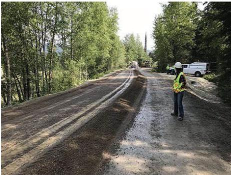
Roads can be raised to remain passable in the event of flooding, sea-level rise, and storm surge. Raising/elevating roads is a well-established strategy and has been implemented in many coastal communities. Adequately designed culverts are needed to facilitate the drainage of water under the raised/elevated roads.
