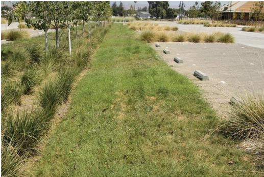
A bioswale is a narrow strip of vegetation that redirects and filters stormwater. It is used to collect runoff stormwater from non-porous surfaces such as roads, parking lots, and rooftops. Bioswales improve water quality by infiltrating the first flush of stormwater and filtering secondary runoff.
