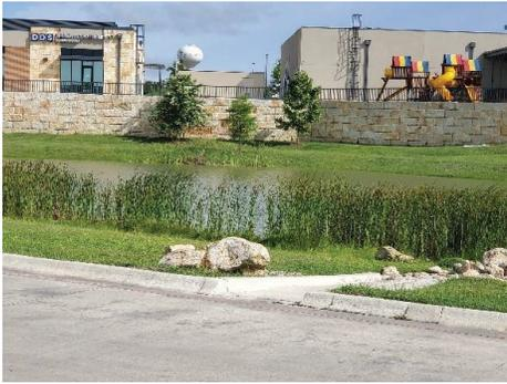
Creating retention and detention ponds is an effective method for managing stormwater by collecting stormwater and releasing it at a rate that prevents flooding or erosion. The main difference between the two is that retention ponds hold water indefinitely, while detention ponds act as a temporary area for storing stormwater. Often, detention ponds are smaller than retention ponds.
