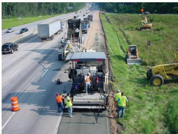
Enhancing or hardening (i.e., providing additional lateral support for) paved shoulders can reduce the damage to the pavements and roads from inundation and storm surge in some circumstances.
