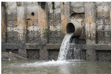
A culvert "conveys surface water through a roadway embankment or away from the highway right-of-way (ROW) or into a channel along the ROW."<sup>ii</sup> Cleaning and regular maintenance of culverts ensures optimal flow of water through the stormwater management system. A proactive culvert maintenance strategy is effective in helping protect road infrastructure in a flooding event.
