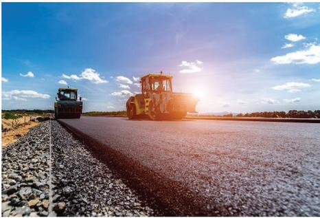
Enhancing the surface of a roadway typically involves additional thickness of the surface course (e.g., 6-inch asphalt layer as opposed to a 4-inch asphalt layer).
