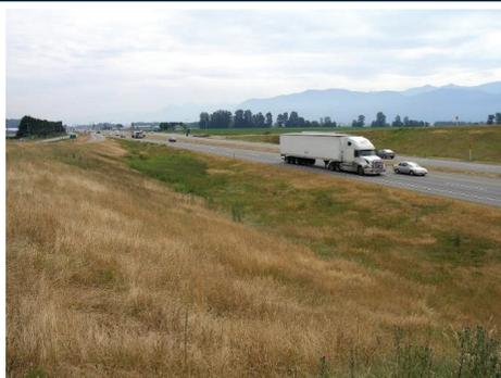
Raised medians are curbed sections that typically occupy the center of the roadway. Depressed medians have a common ditch or swale between divided roadways.
