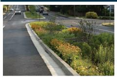
Impervious streets, parking lots, and sidewalks increase peak flow and reduce the time between storm occurrence and peak flow rate. Both factors result in increased localized flooding. Green infrastructure is a stormwater management approach that incorporates vegetation, soil, and engineered systems (e.g., tree wells and biofiltration gardens) to slow, filter, and clean stormwater.
