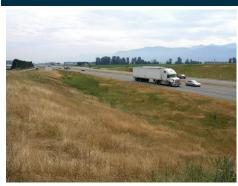
Raised medians are curbed sections that typically occupy the center of the roadway. Depressed medians have a common ditch or swale between divided roadways.
