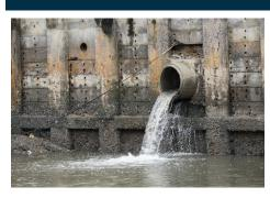
A culvert "conveys surface water through a roadway embankment or away from the highway right-of-way (ROW) or into a channel along the ROW." Cleaning and regular maintenance of culverts ensures optimal flow of water through the stormwater management system. A proactive culvert maintenance strategy is effective in helping protect road infrastructure in a flooding event.
