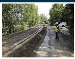
Roads can be raised to remain passable in the event of flooding, sea-level rise, and storm surge. Raising/elevating roads is a well-established strategy and has been implemented in many coastal communities. Adequately designed culverts are needed to facilitate the drainage of water under the raised/elevated roads.
