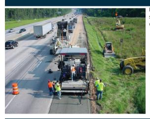
Enhancing or hardening (i.e., providing additional lateral support for) paved shoulders can reduce the damage to the pavements and roads from inundation and storm surge in some circumstances.
