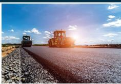
Enhancing the surface of a roadway typically involves additional thickness of the surface course (e.g., 6-inch asphalt layer as opposed to a 4-inch asphalt layer).
