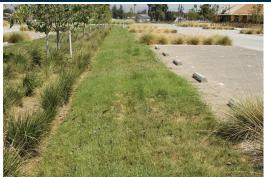
A bioswale is a narrow strip of vegetation that redirects and filters stormwater. It is used to collect runoff stormwater from non-porous surfaces such as roads, parking lots, and rooftops. Bioswales improve water quality by infiltrating the first flush of stormwater and filtering secondary runoff.
