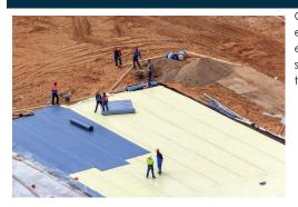
Geosynthetics/geotextiles (such as green mats) are increasingly used in strengthening or enhancing the resiliency of transportation infrastructure. Geotextiles/Geonets are used to enhance drainage, Geogrids and geotextiles are typically used on embankments and to strengthen pavement layers, and geotubes and erosion control mats are used effectively to mitigate beach erosion.
