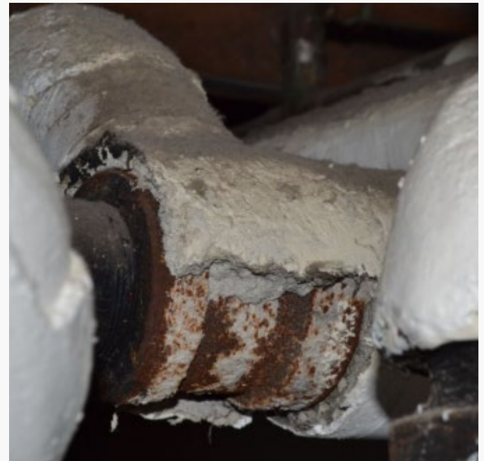
Asbestos pipe wrap (joint partially removed) (EPA website)
