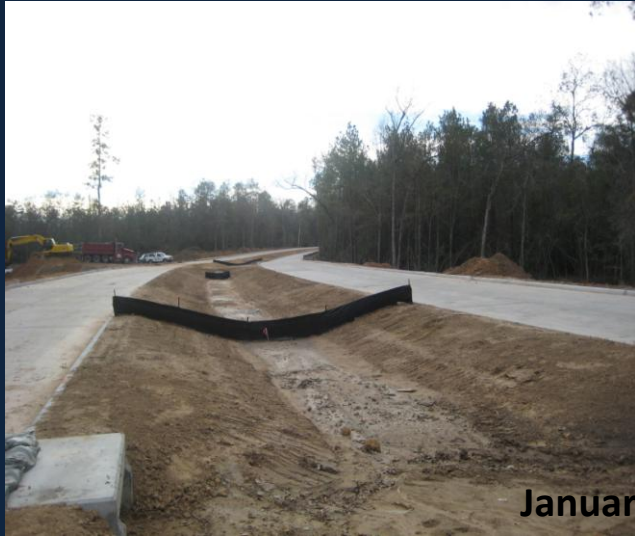
Center median bioswale, false curb inlets, berms, riprap
