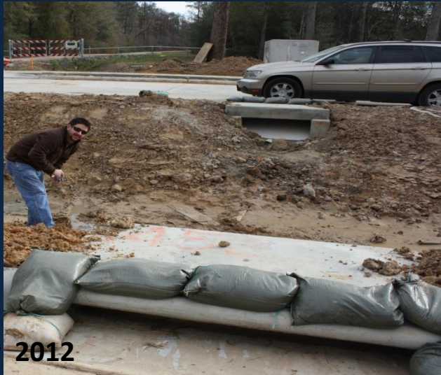
Center median bioswale, false curb inlets, berms, riprap
