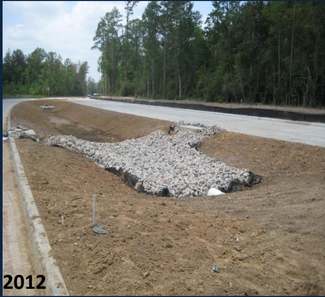
Center median bioswale, false curb inlets, berms, riprap
