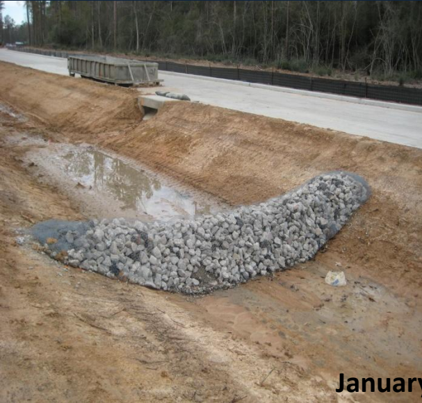
Center median bioswale, false curb inlets, berms, riprap
