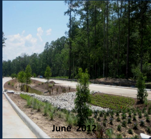
Center median bioswale, false curb inlets, berms, riprap
