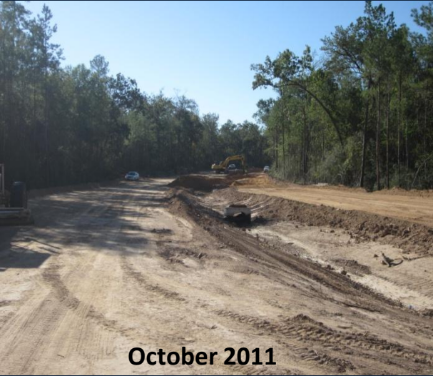
Center median bioswale, false curb inlets, berms, riprap
