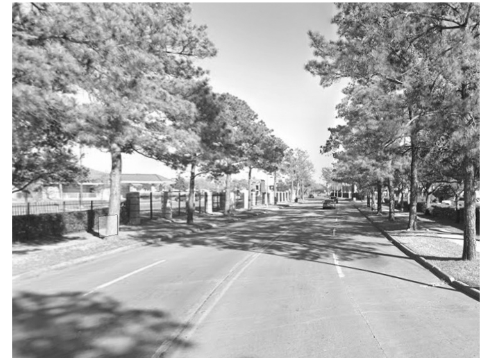
The existing four lane design on Creekbend Drive makes bicycling uncomfortable for most people.
