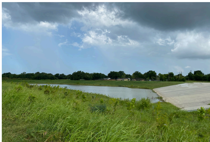
New areas of flooding have emerged in recent years.
