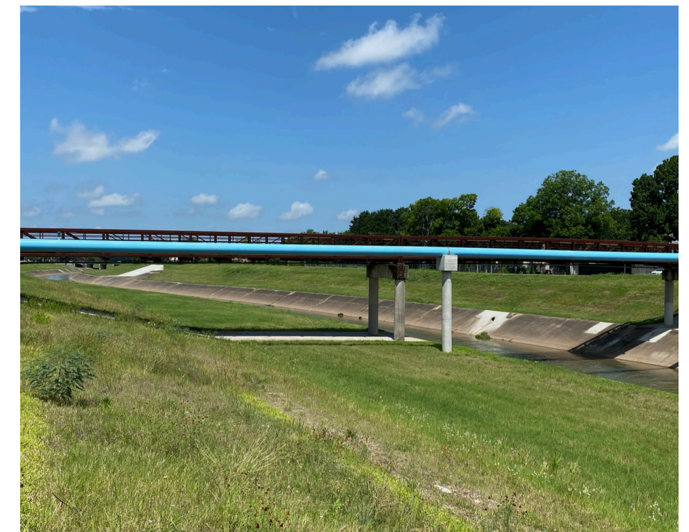
Sanitary sewer line as seen in the study area.
