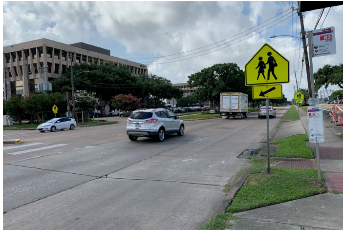
Crosswalks and striping needs maintenance. Bike paths are missing.
