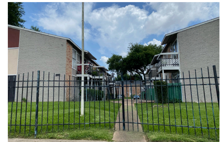
Access to pedestrian facilities and bayous could be improved.
