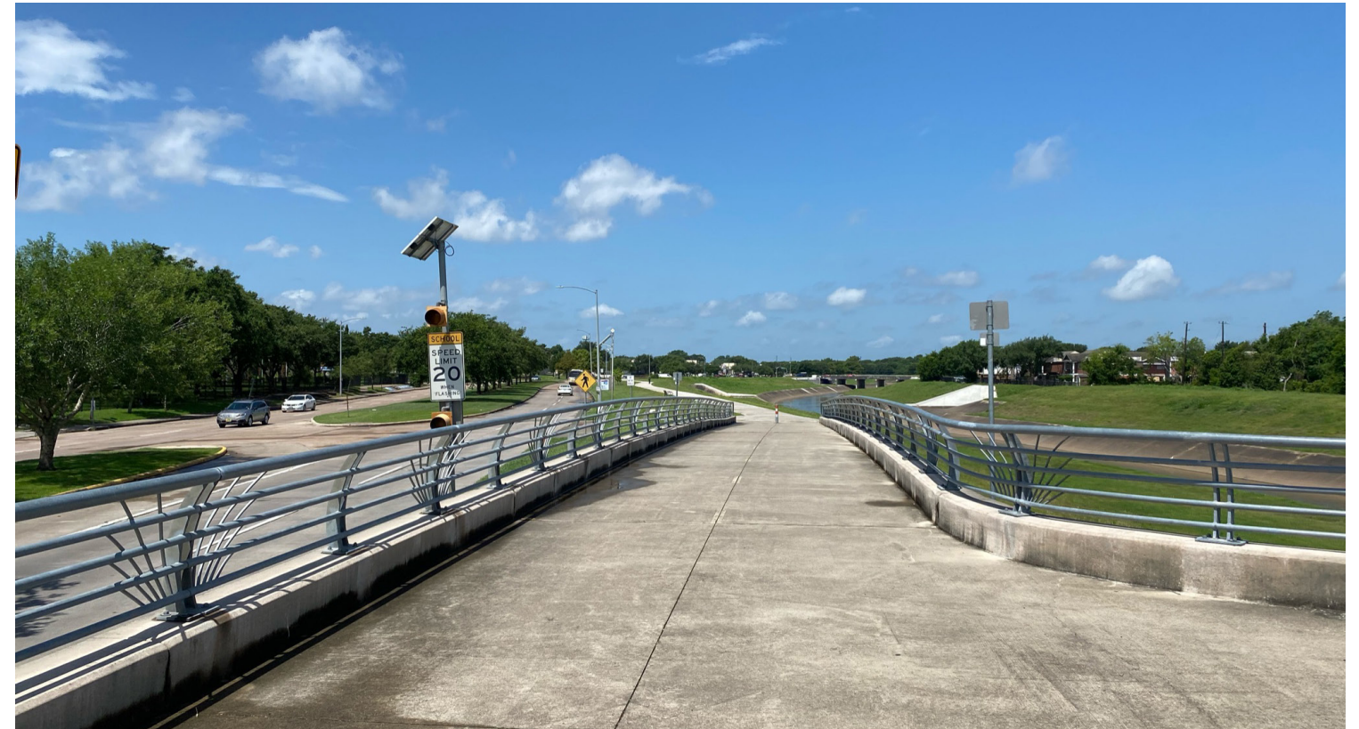
A bike path separated from the street provides a higher level of comfort for the cyclist.
