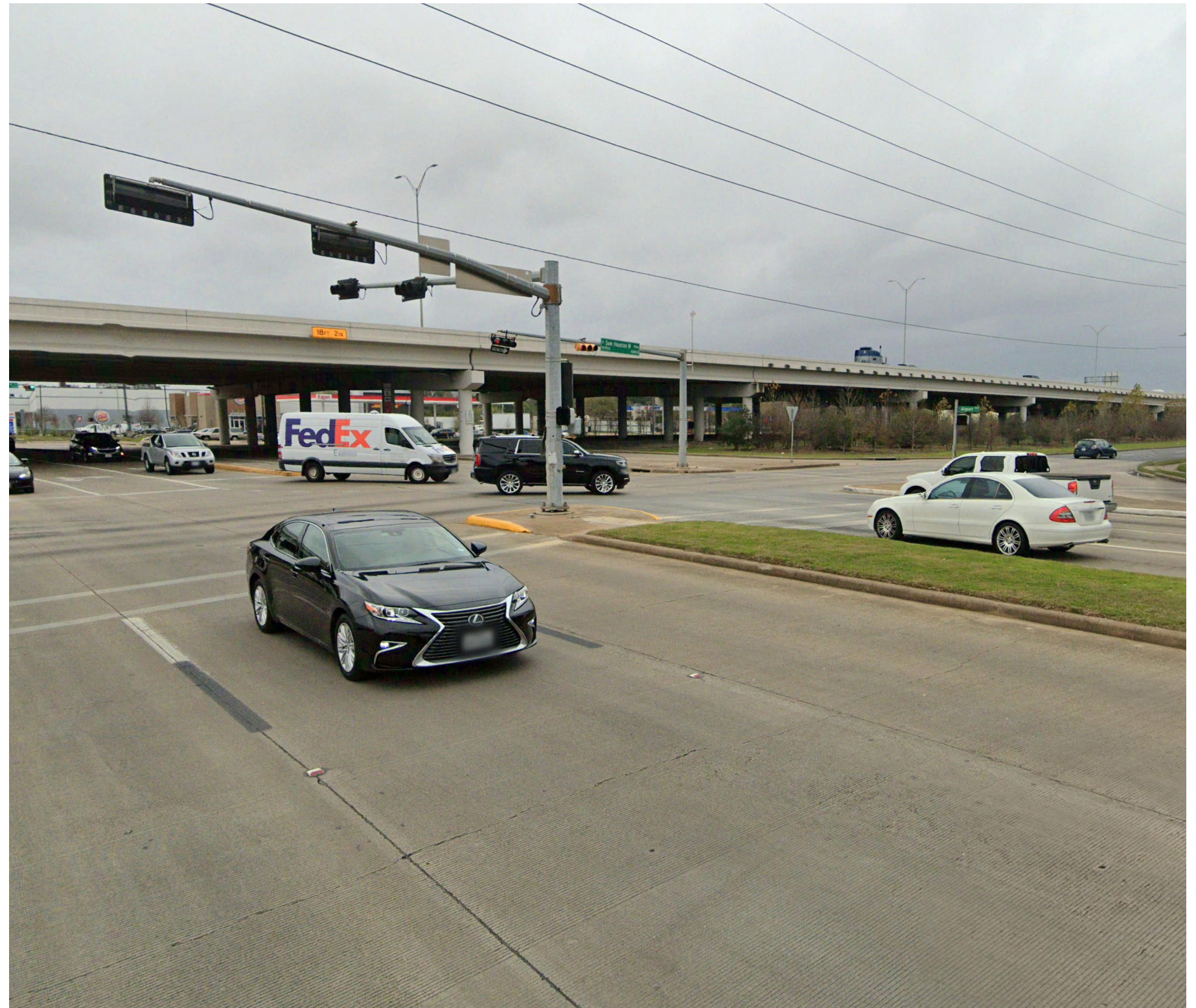
Intersection at Sam Houston Parkway and West Bellfort Avenue is a good location for gateway markers.
