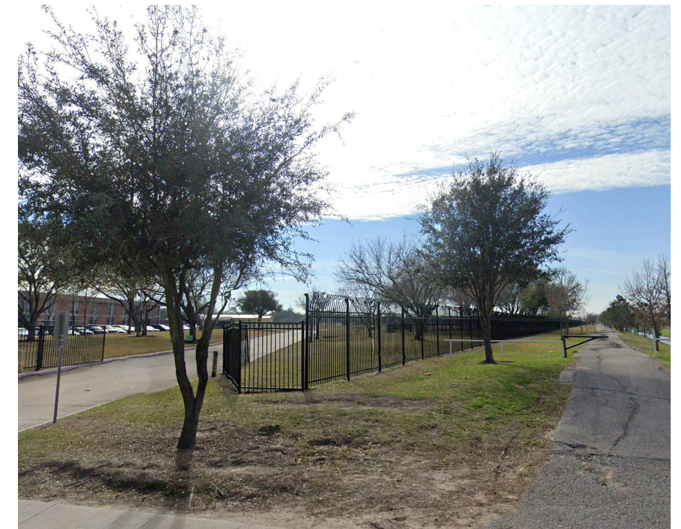
There is a poor connection between the Bayou and Fondren Middle School.
