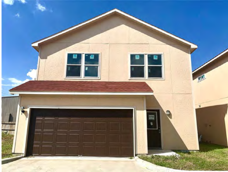
Figure 9: Example of New Construction in Brays Oaks
