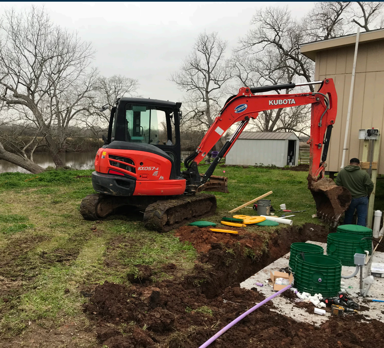
PHOTO: Installation of a new aerobic On-Site Sewage Facility in Brookshire (Waller County)
