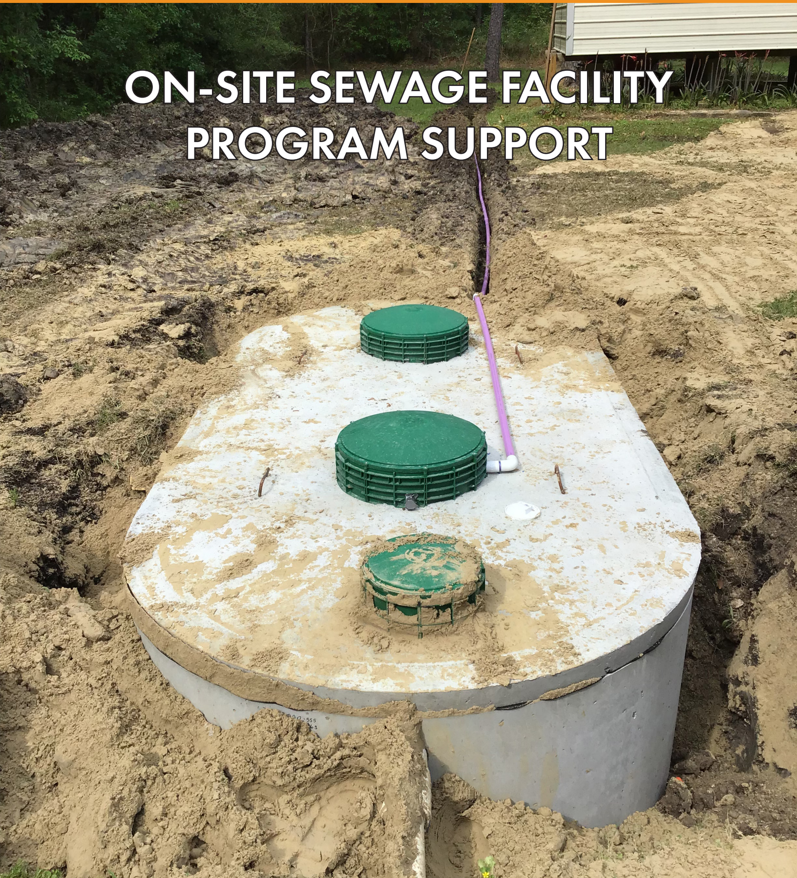
PHOTO: Installation of new aerobic On-Site Sewage Facility
