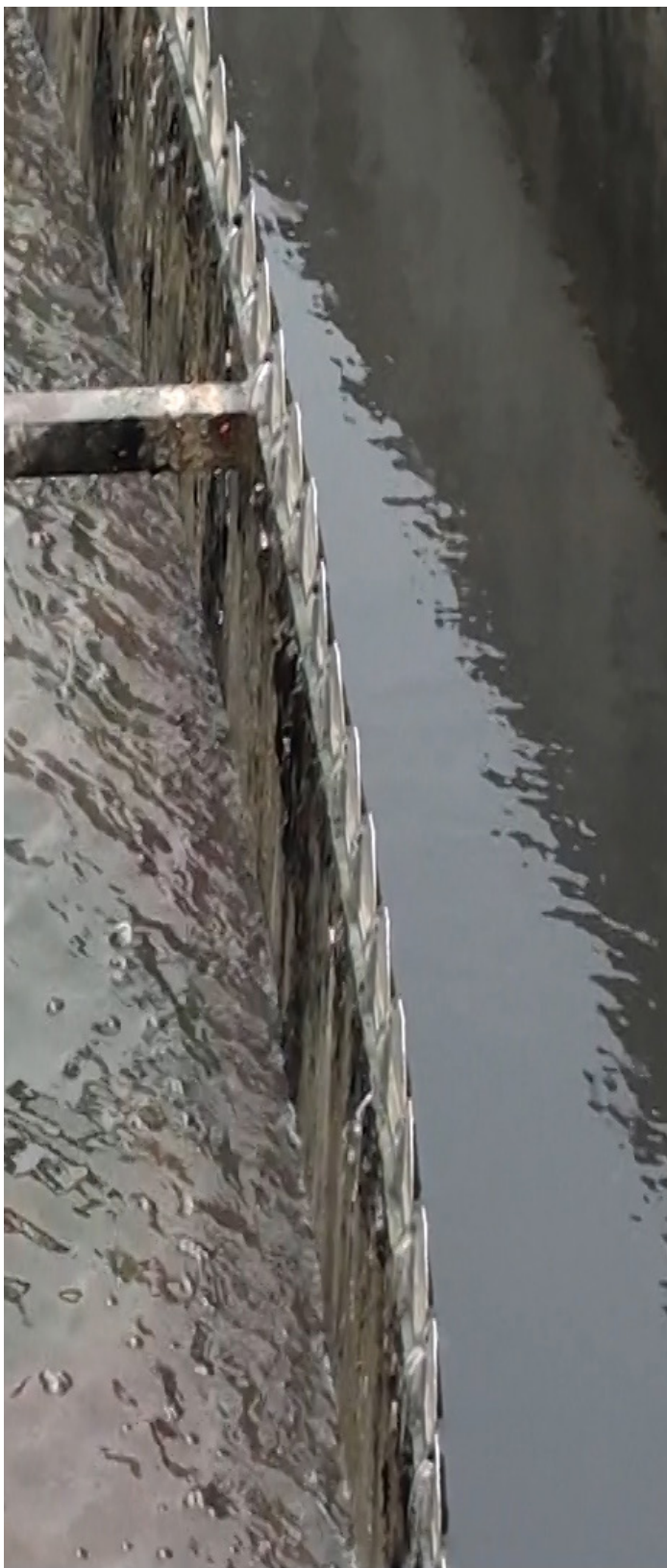
PHOTO: Saw-tooth weir, League City Wastewater Treatment Facility
