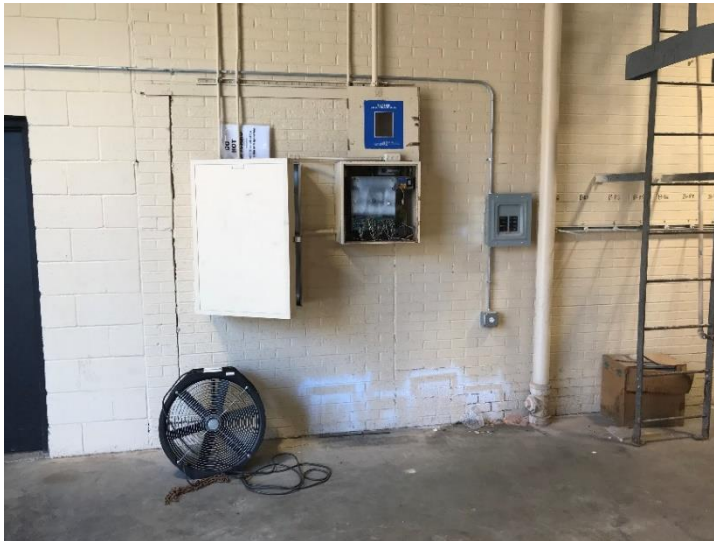
Figure 2-13 Selected Vehicle Storage Locations With Power Supply Provisions to Connect Battery Charging Equipment
