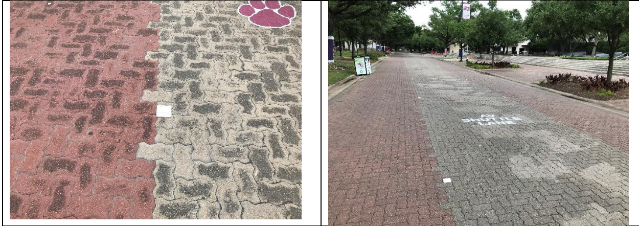
Figure 2-11 Reflective Markers and Colored Tile to Designate the Dedicated AV Shuttle Lane
