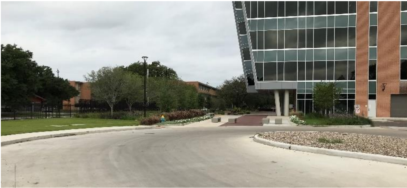
TSU Station Next to TSU Library at the East End of the Tiger Walk Pedestrian Facility
