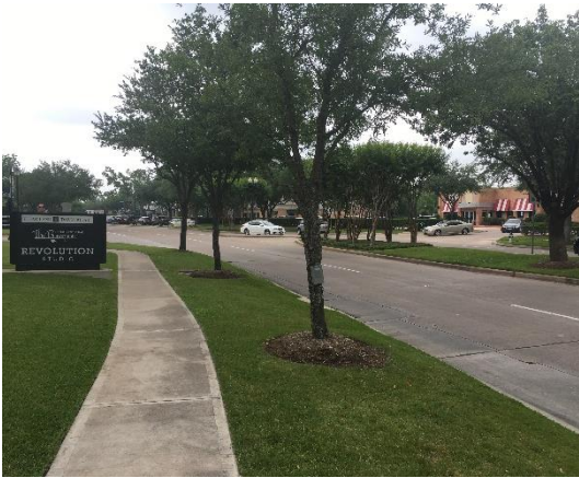
Image 1: Sidewalk along Town Center Boulevard Southbound at Texas Drive Facing North
