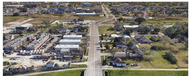
On Vista Looking East: Bayou Trail at Grade Crossing
