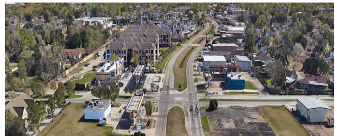
On Fairmont Looking East: Bayou Trail at Grade Crossing
