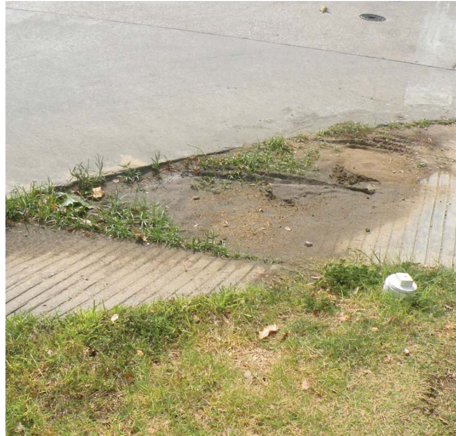
Improper grading and construction details leads to maintenance hassles.
