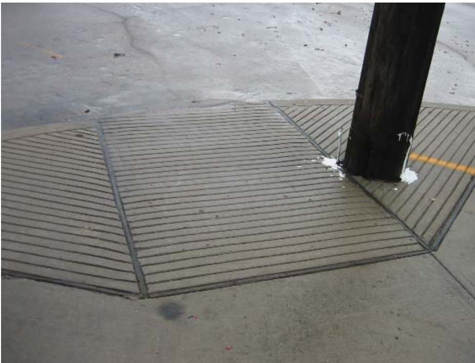
Previously ADA compliant ramps do not have the truncated domes that are required by new ADA standards.
