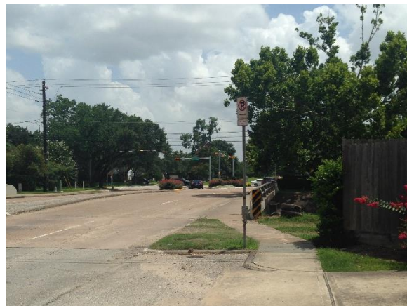
Image 6: Sidewalk along S. Rice Ave. Facing South
