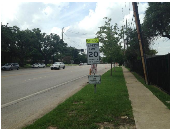
Image 1: Sidewalk along S. Rice Ave. Facing North
