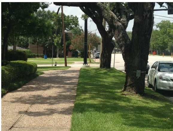
Image 3: Sidewalk along S. Rice Ave. Facing North
