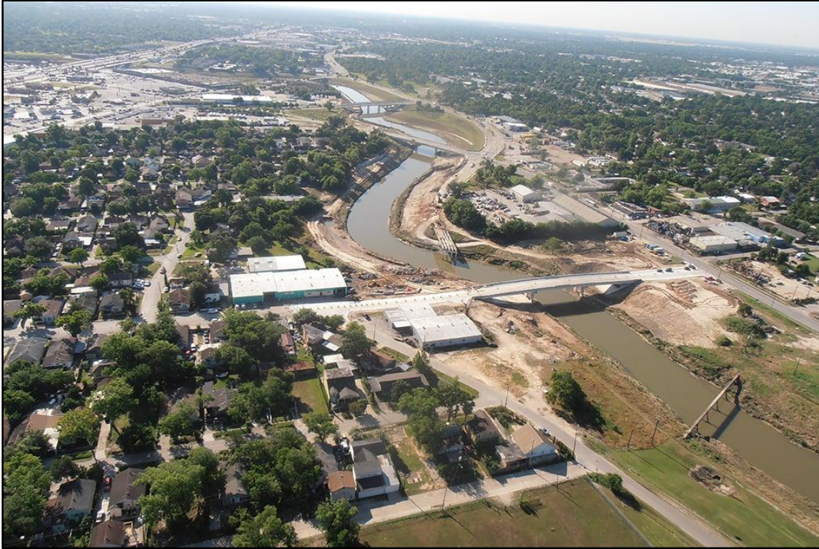
Figure 16. Photo showcasing modifications to a bridge on Brays Bayou to allow for increase in bayou flow. Photo courtesy of Harris County Flood Control District.
