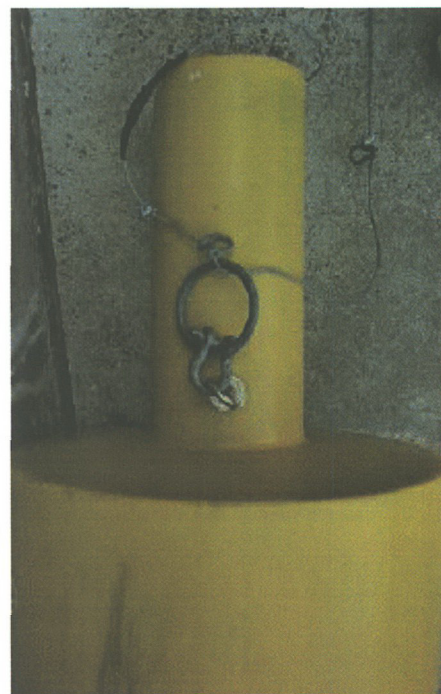
Photo 12 - Four inch (4") galvanized ring attached to "eye" of buoy.
