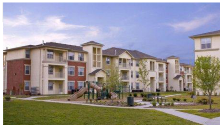
Costa rialto housing development
