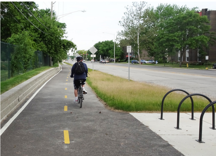
Shared-use paths allow bicyclists and pedestrians to safely travel along roadways without interfering with vehicle traffic Source: Burke Engineering
