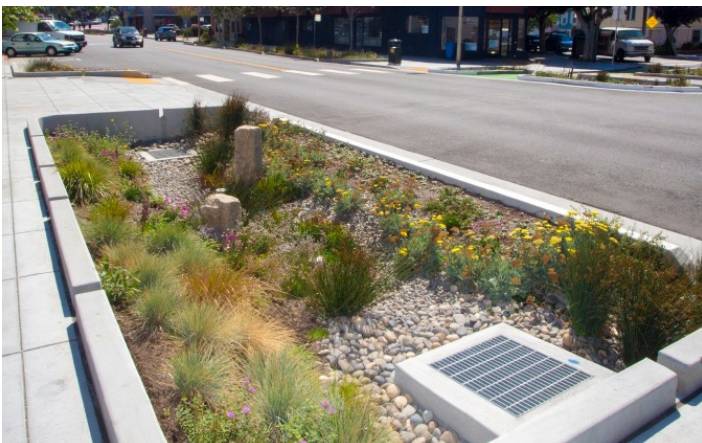
Green infrastructure can be incorporated along roadways and help filter water runoff Source: Lotus Water
