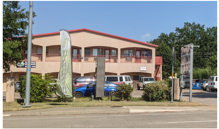
Existing retail and apartments along Sandra Bland Parkway Source: Half
