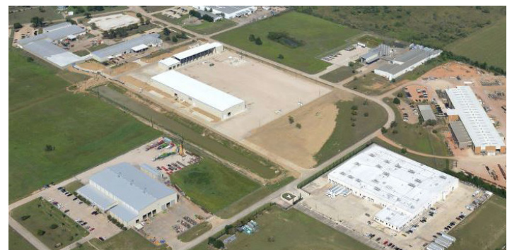
Waller Industrial Park at GH Circle Source: Archway Properties
