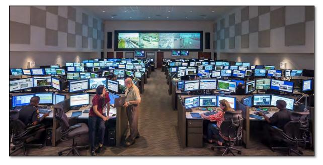
The Houston region (including the US 59/IH-69 corridor) has an extensive deployment of ITS infrastructure. The hub for the monitoring and control of the infrastructure is Houston TranStar, the multi-agency regional transportation and emergency response center. Freeway, tollway and managed lane operations are all monitored from Houston TranStar using the ITS infrastructure.
