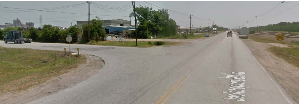
Figure 2.5 Jacintoport Blvd. at Appelt Dr. - Looking East
