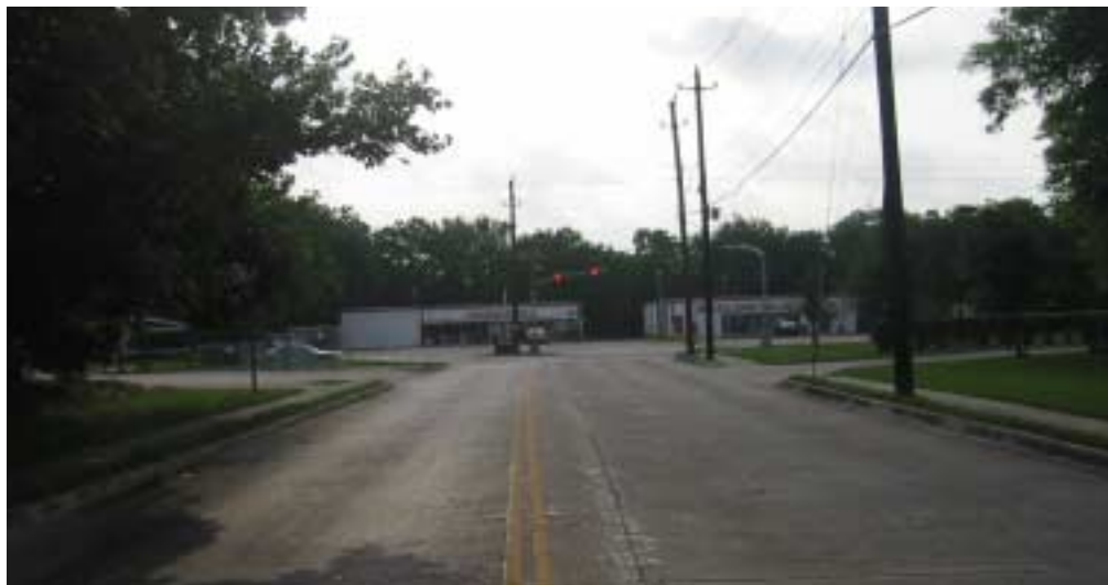
Figure 15. View of Preston @ Cherry Brook from the Eastbound Approach.
