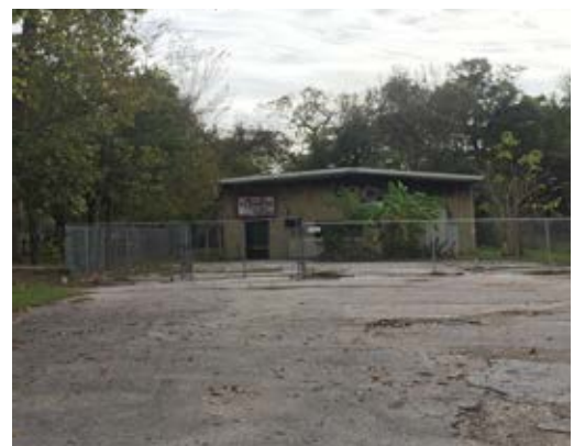
Environmental hazards are a problem that needs to be addressed.
