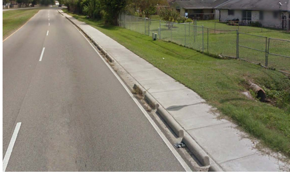
Sidewalk constructed along an open ditch roadway in Houston, TX
