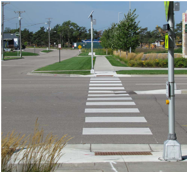
Visible crosswalk with pedestrian-only signal
