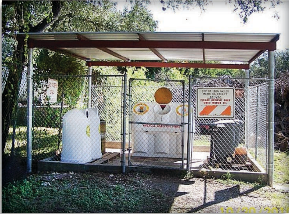
The used oil recycling container is available 24/7 and holds 400 gallons. Yearly collection averages 2,500 gallons, which might otherwise have been illegally dumped.
