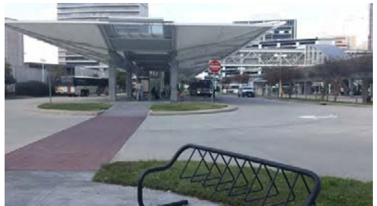
Figure 5.143: Crosswalk leading from bike racks to boarding area
