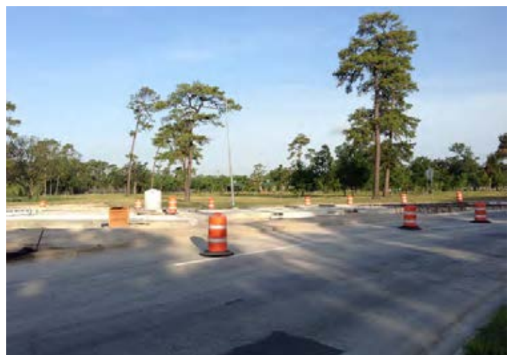
Figure 5.98: METRORail station under construction; little activity adjacent to the site
