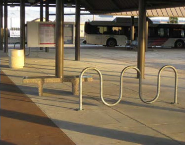
Figure 5.59: Existing bike racks under canopy
