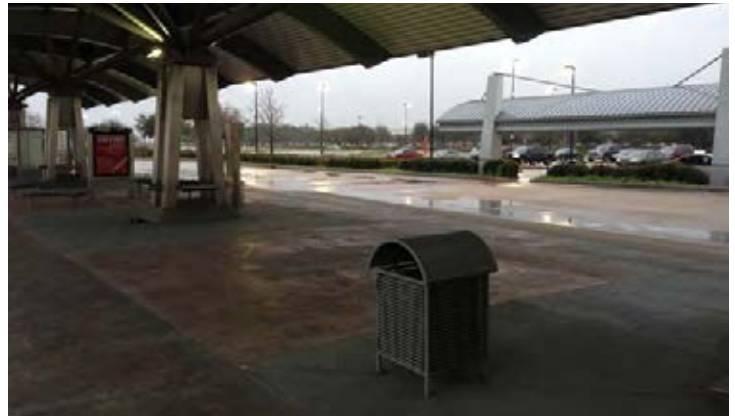
Figure 5.166: Space under the boarding area canopy
