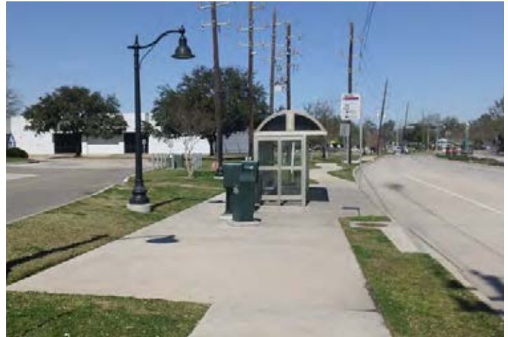
Figure 5.72: The Greenspoint Transit Center has two bus shelters located along Greenspoint Drive
