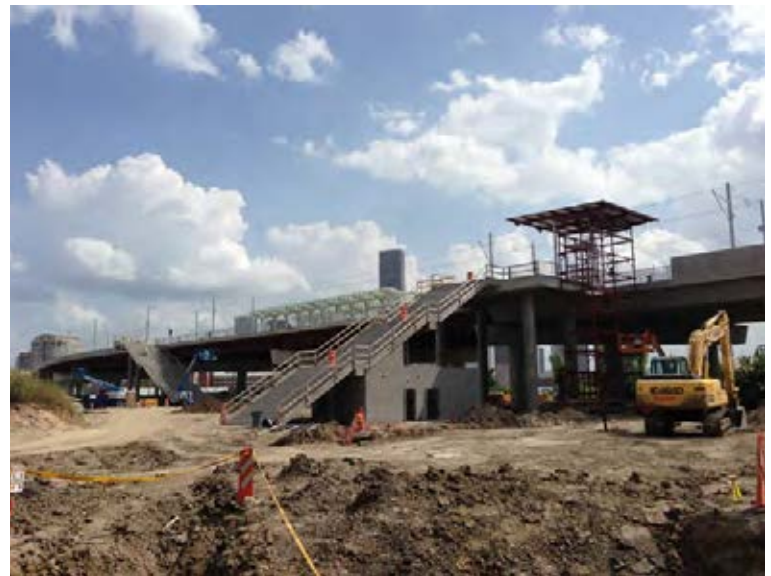
Figure 5.44: Staircase from station to future Transit Center
