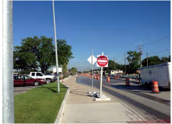
Figure 5.129: Eastbound bus bay with platform on the right
