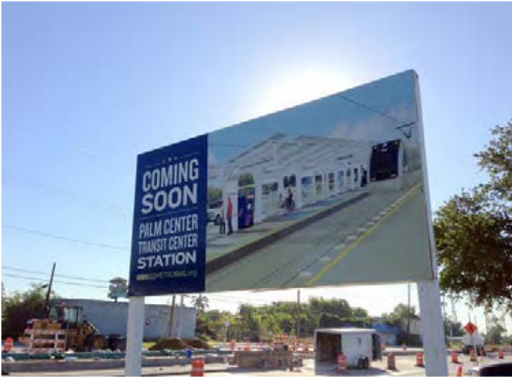
Figure 5.128: Sign announcing future station with platform in the background
