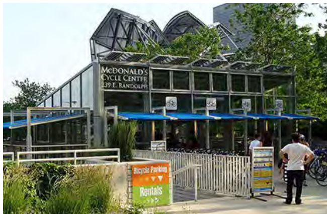
Figure 5.17: Exterior of McDonald's Cycle Center at Millennium Park in Chicago Photo: treehugger.com
