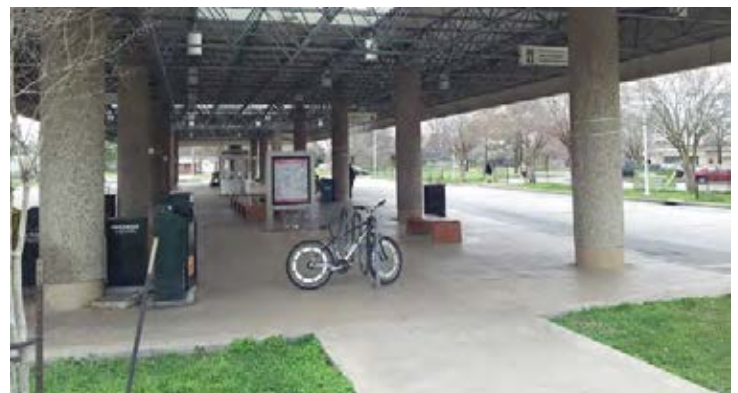
Figure 5.89: Bike locked to bike rack under Transit Center canopy
