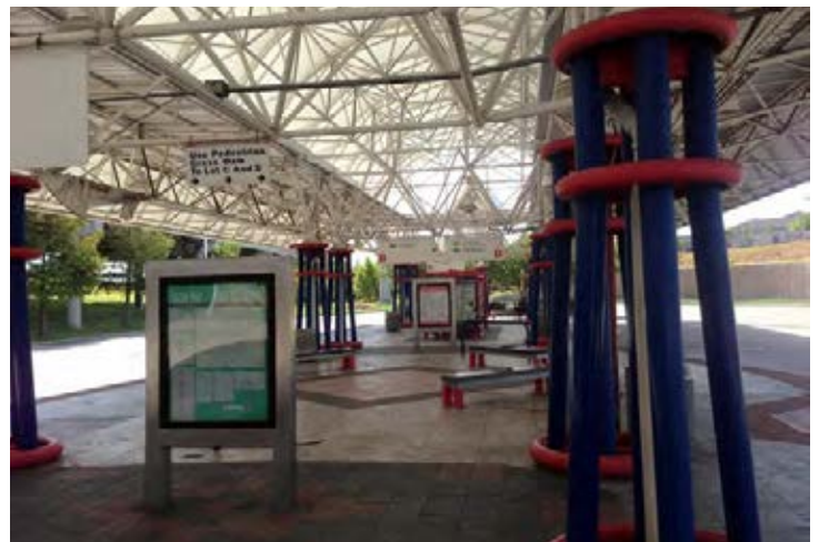
Figure 5.161: Space under canopy that could potentially be used for bike racks
