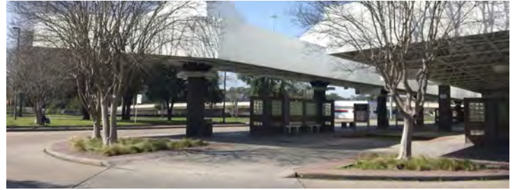
Figure 5.122: Ramp to Transit Center from the parking lot
