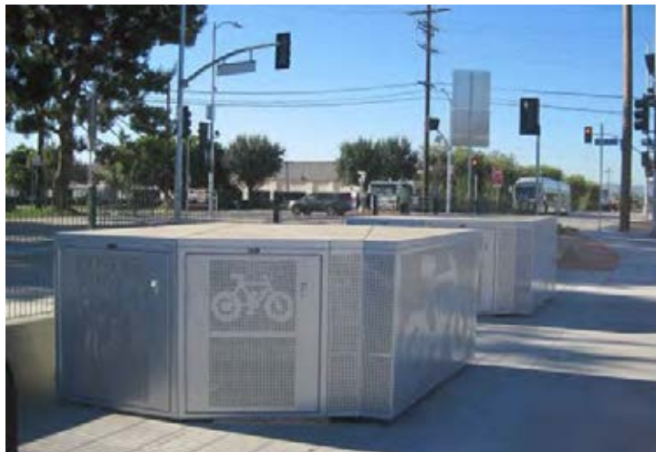
Figure 4.15: Los Angeles Metro bike lockers Image credit: thesource.metro.net
