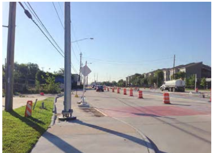
Figure 5.130: Westbound bus bay with station entrance to the right
