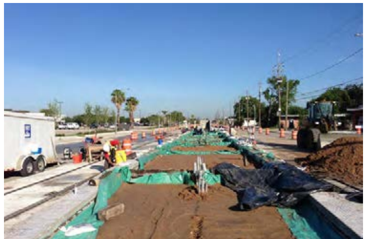
Figure 5.131: Light rail platform under construction
