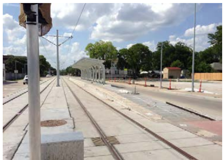
Figure 5.134: Quitman Station under construction
