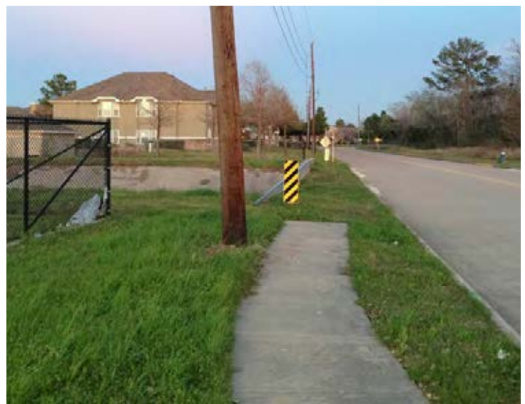
Figure 5.117: Sidewalk ends at the edge of METRO property and does not reach nearby apartments
