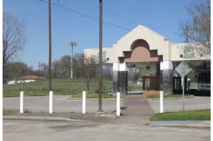
Figure 5.22: Ramp to boarding area from driveway loading area
