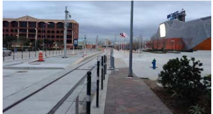
Figure 5.55: Future METRORail station adjacent to Dynamo Stadium
