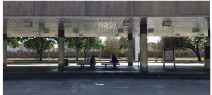
Figure 5.81: There is enough space under the cover of the Hiram Clarke Transit Center for bike parking facilities, which should be placed in a way that won't obstruct circulation
