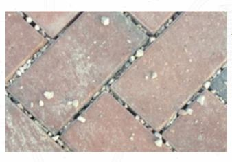
Pervious Pavers – Aggregate needs added
