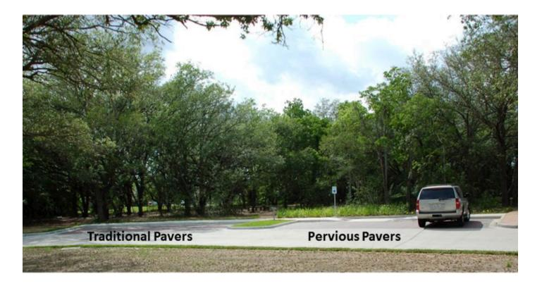
The pervious pavers are designed with small spaces between each paver so water can seep down between the stones and into the gravel base below. Water can then either soak into the soil or drain into a perforated pipe located below ground. This pipe is connected to the storm drain system.
