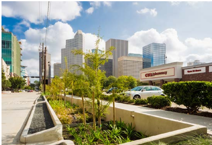
BAGBY STREET bioretention
