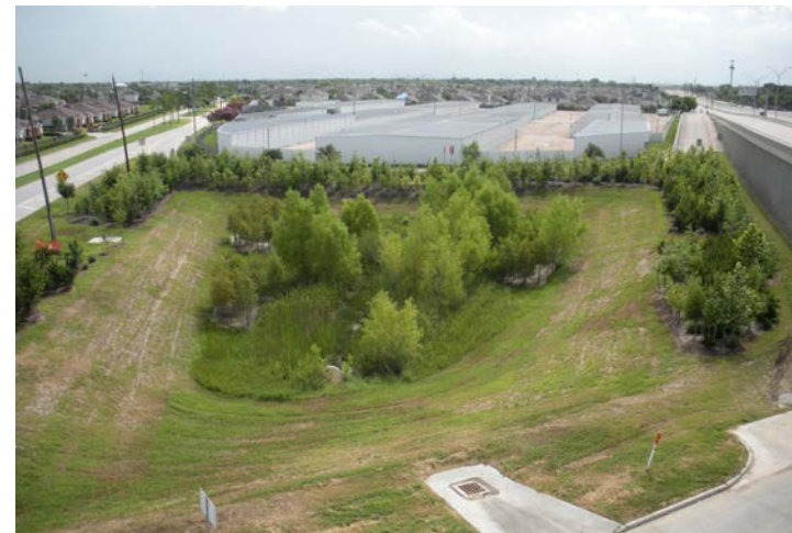
WESTPARK TOLLWAY bioretention
