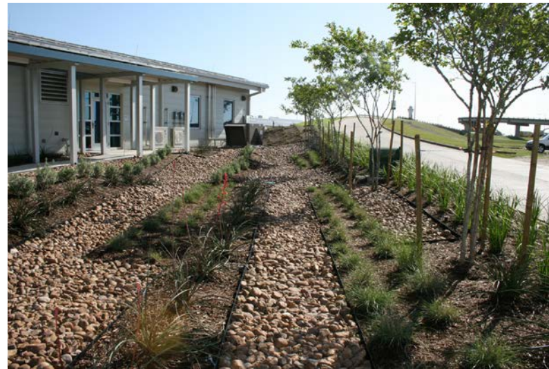
IAH CONTROL BLDG bioretention
