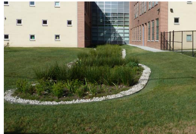
PECK ELEMENTARY bioretention
