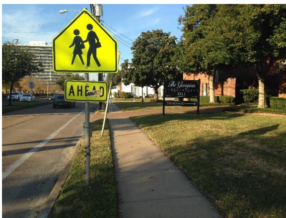
Image 9: Sidewalk along Willowick Road Facing North
