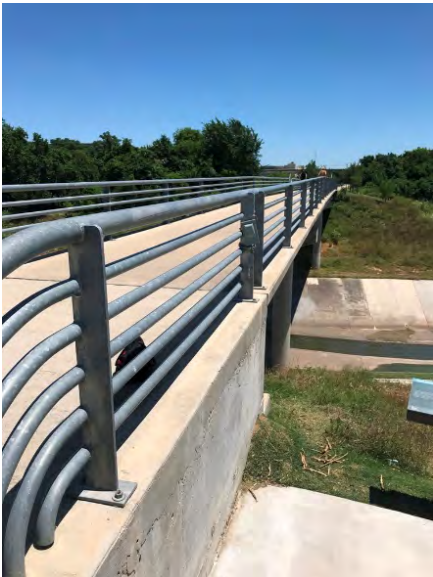
Image 1: Bridge over White Oak Bayou (looking east)
