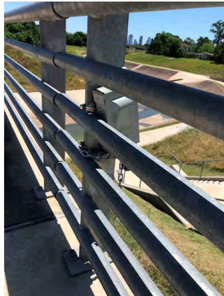
Image 2: Bridge over White Oak Bayou (zoomed)
