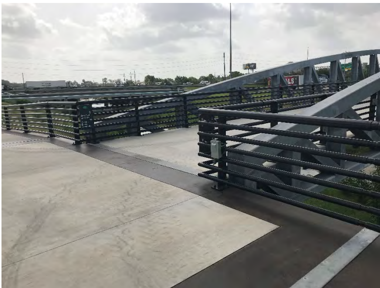
Image 1: Path by pedestrian bridge (looking west)
