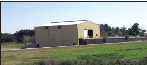
City of Huntsville Transfer Station
