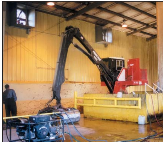
City of Huntsville Transfer Station
