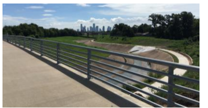
New Segment of White Oak Trail Under Construction
