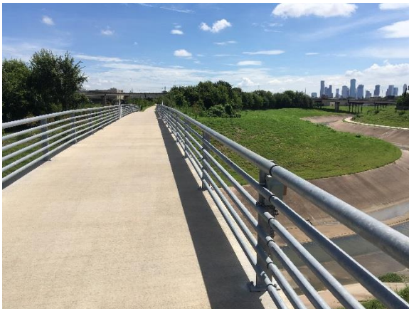
Image 13: Bridge over White Oak Bayou Facing East
