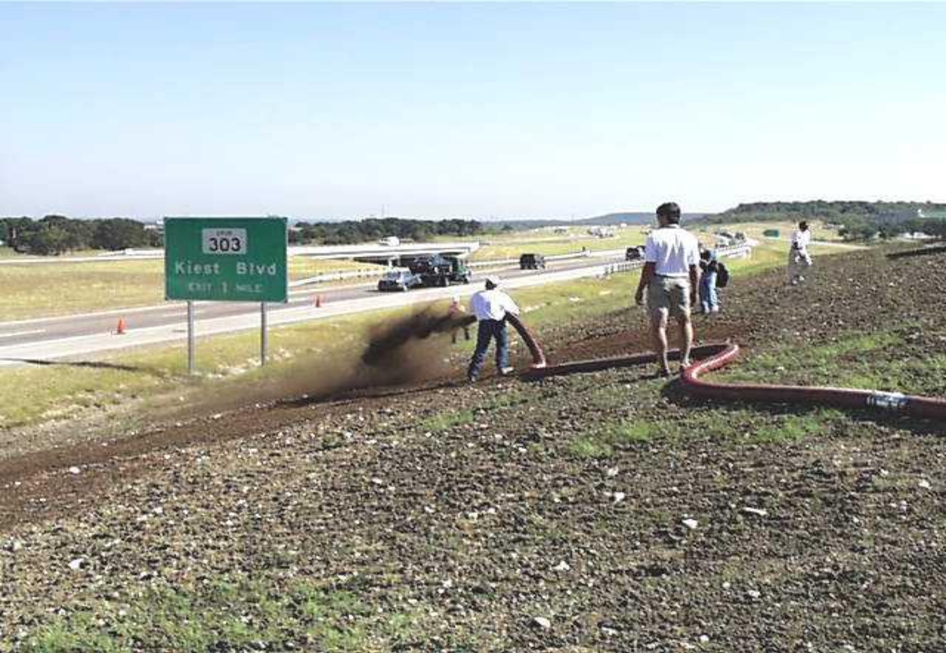
Dallas/Spur 408 Demonstration August 1999
