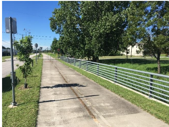
Image 14: Columbia Tap Trail at Polk Street Facing South
