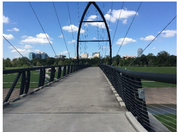
Image 38: Bill Coats Bridge at Hermann Park Facing West
