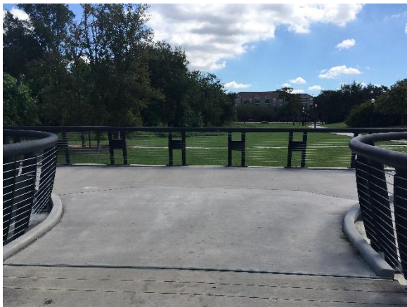
Image 37: Bill Coats Bridge at Hermann Park Facing East
