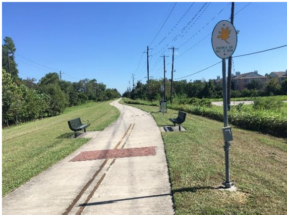
Image 23: Columbia Tap Trail at North MacGregor Way Facing North
