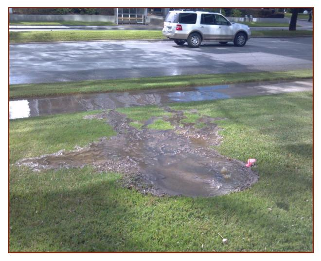
Figure 3 - Sanitary Sewer Overflow (SSO) near Greenway Plaza, Houston, TX
