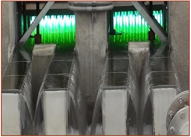
Figure 8 – UV disinfection of wastewater effluent
