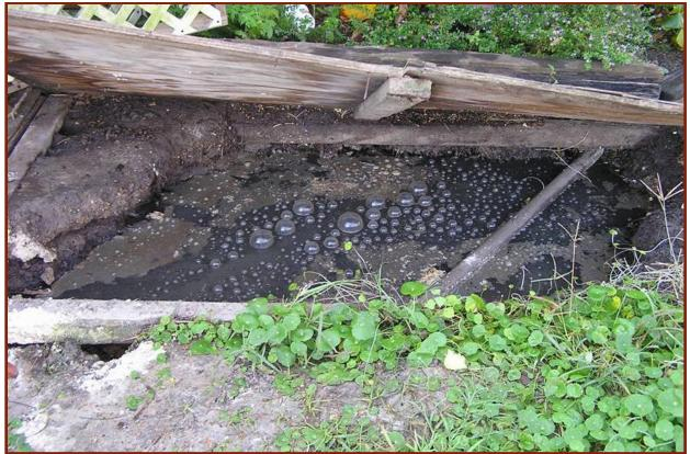
Figure 11 - Discharge from failing OSSF
