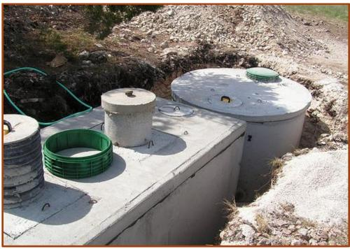
Figure 13 - Installation of an OSSF
