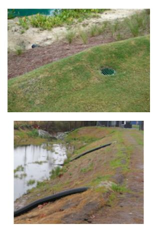
Figure 15. Two examples of using slope drains for bank stabilization. Surface water generated during larger storms flowing into the wetland is directed into the drains. The drainage reduces erosion that would result from concentrated flow down the banks.
