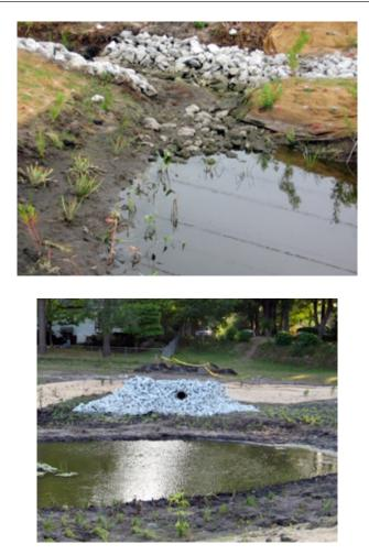
Figure 16. Use riprap of granite or marl to slow inflow to the wetland and protect the inlet from erosion.
