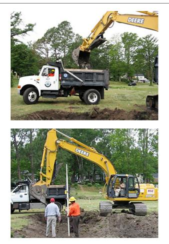
Figure 11. Keep dump trucks moving for off-site transport of soil (top), and keep the excavator operator updated on correct grade to speed construction (bottom).
