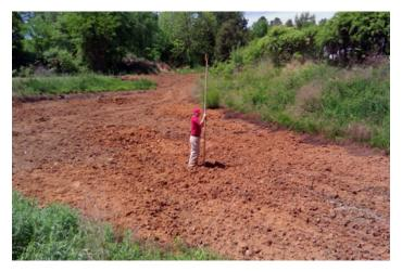
Figure 13. Surveying a properly prepared wetland surface.
