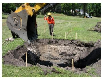
Figure 3. Stake out the wetland perimeter, internal wetland features, and locations of structures prior to excavation. Make sure all existing utilities at the site are located and marked.
