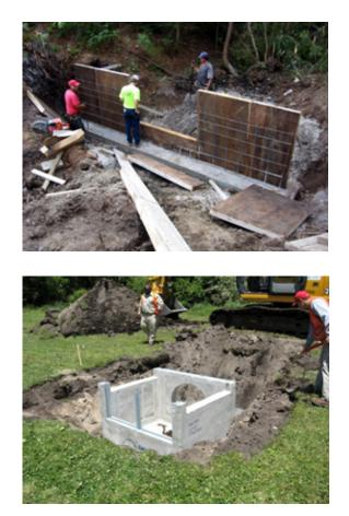
Figure 8. Examples of outlet structures built onsite (*top*) and prefabricated and delivered to the site (*bottom*)
