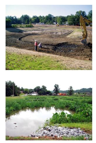
Figure 19. Adding features and topsoil in a large wetland. Side-slopes have already been prepped, and grass is coming up (top). After 1 year, vegetation is successfully established (bottom).
