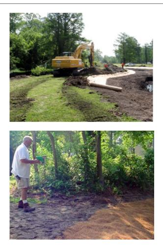
Figure 14. Stabilize banks daily with lightweight fabric and seeding to reduce the chance of erosion while the wetland develops.
