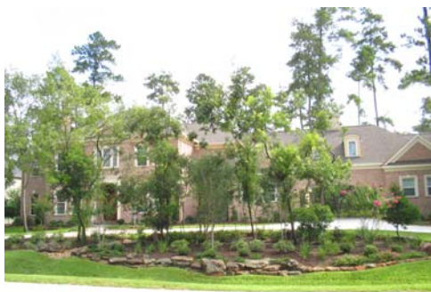
Figure 88. House Two at completion
