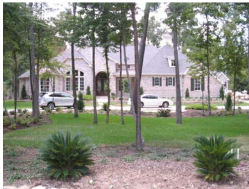
Figure 45. Completed House One
