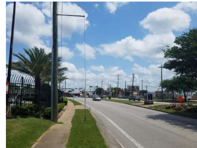
Looking East at Wirt along WB Kempwood
