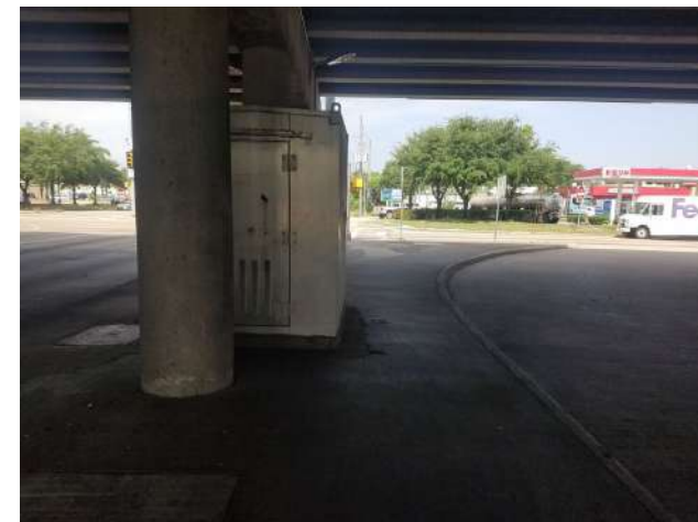
North side — traffic box choke point: 6' to U-turn
