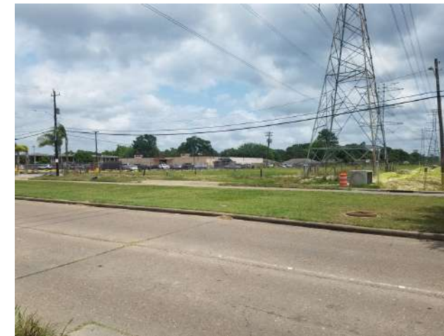
CenterPoint easement crossing at Mangum
