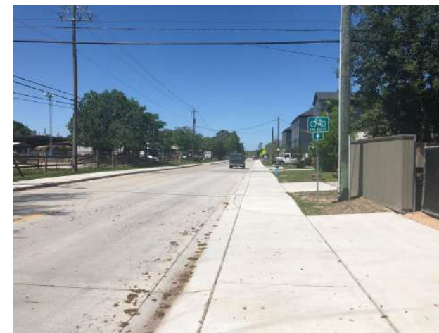
Newly Constructed Sidewalk & Roadway
