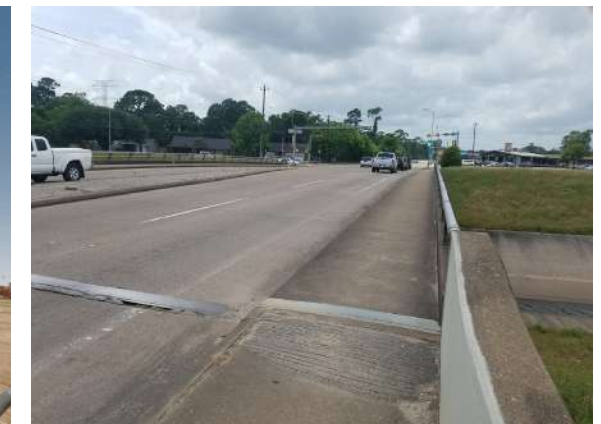
34th St bridge looking west
