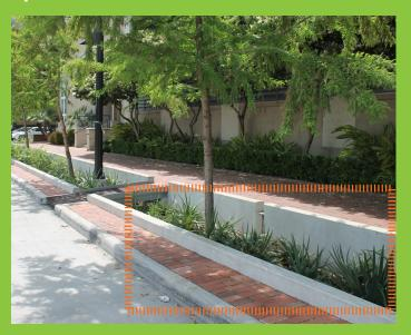
A bioretention area is an upland soil and plant-based filtration mechanism designed to control and improve the quality of stormwater runoff. A properly designed bioretention area can infiltrate and temporarily store runoff, reducing a site's overall runoff volume and helping preserve predevelopment peak discharge rate and timing. Bioretention areas are proven to reduce pollutant loads. There are two main types of bioretention systems: bioretention cells and tree box filter.
