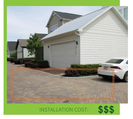
Permeable pavement is designed to allow water to pass through the surface into the soil or underdrain/ subsurface detention or retention system. These systems treat stormwater that falls directly on the surface as well as runoff from adjacent impervious surfaces. Permeable pavement includes a wide range of paved or load-bearing surfaces that can be used as a substitute to conventional pavement on parking areas and low traffic roads (no truck traffic). This technique should
