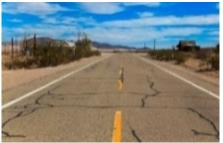
Longitudinal and traverse cracks, occasional patching in good conditions, slight distortions
