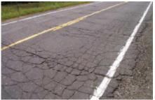
Severe Distortions, Alligator Cracking, Extensive Patching, Potholes
