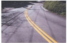
New construction, recent overlay, occasional cracks that are sealed, shows some traffic wear
