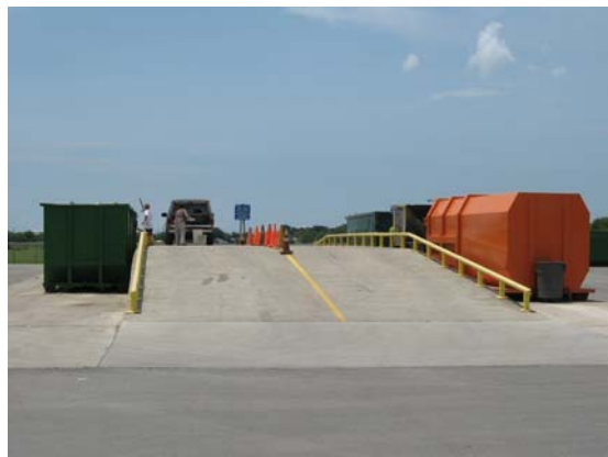
Figure 5-6: Ramp to access roll-offs for household garbage
