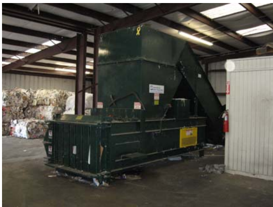
Figure 1-6: Baler inside drop-off facility
