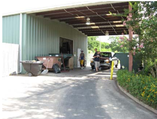
Figure 1-2: Drive-through drop-off area
