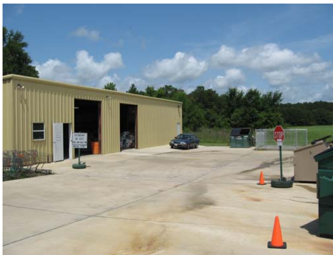
Figure 2-1: Recycling Drop-off Facility
