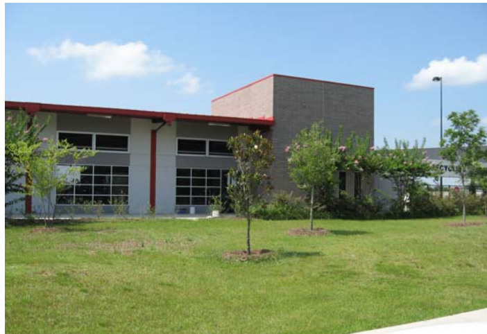
Figure 4-1: Recycling Drop-off Facility
