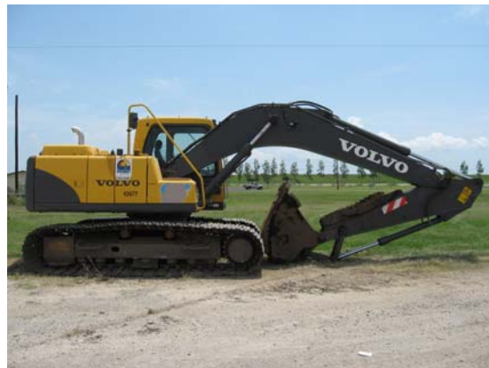
Figure 5-11: Crawler Excavator Used by City
