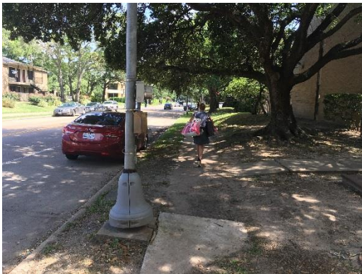
Image 17: Sidewalk along Walnut Bend Lane Northbound South of Richmond Avenue Facing North
