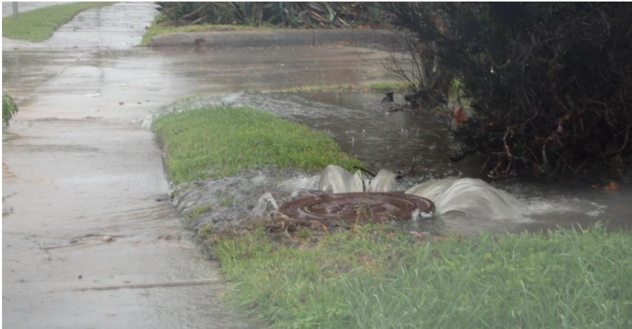
Figure 2 - Sanitary Sewer Overflow following heavy rain event
