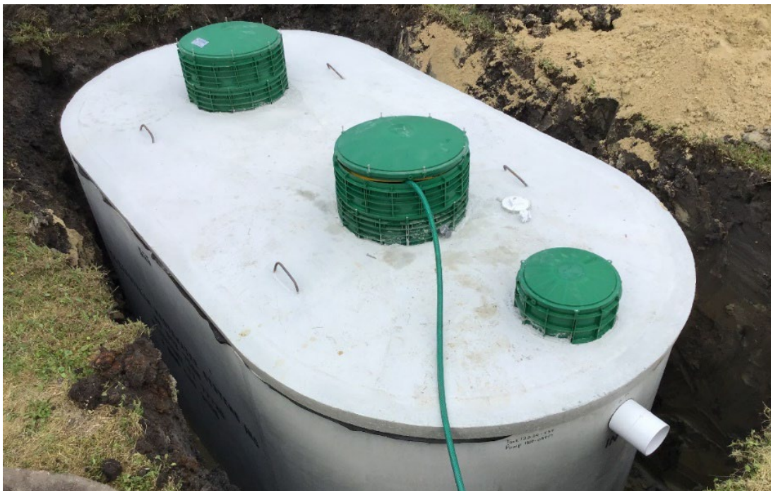
Figure 4 - Installation of an aerobic On-Site Sewage Facility
