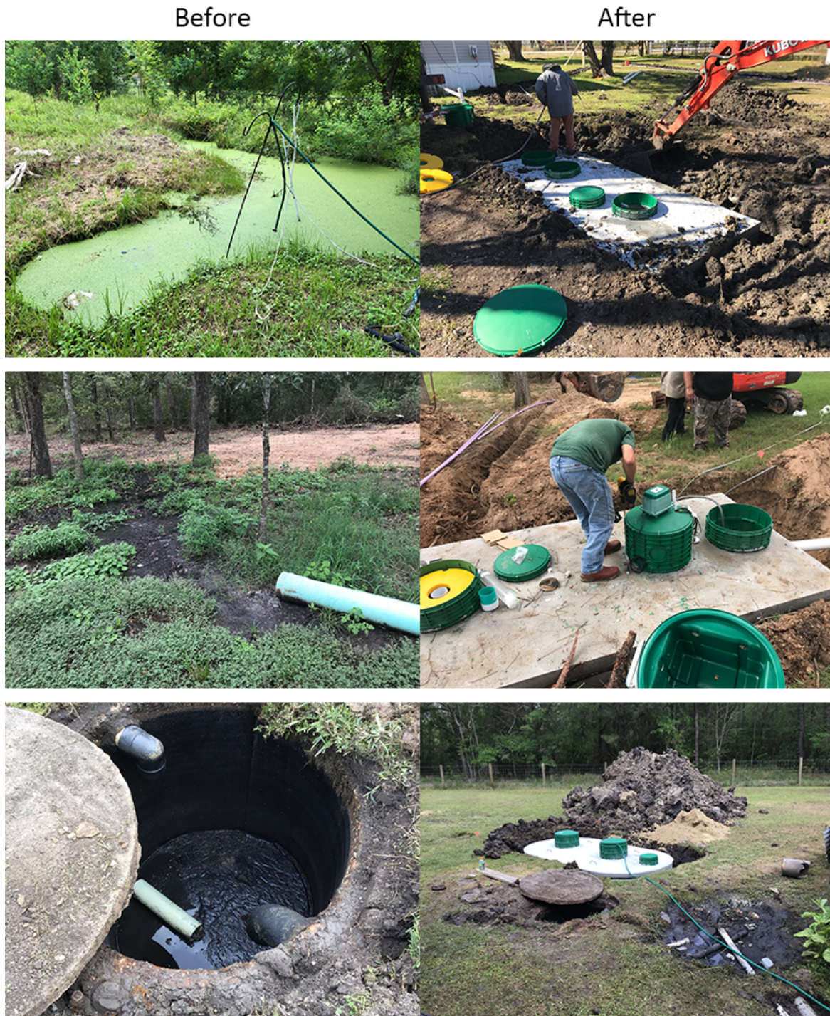
Figure 21 - OSSF Replacement Photographs, Before (Left) and After (Right)
