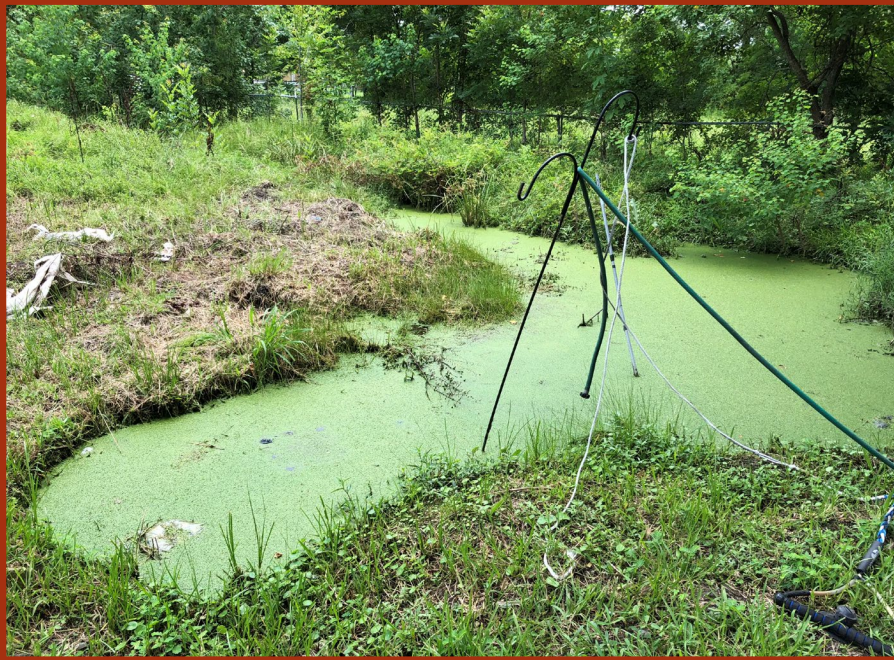
Failing conventional system
