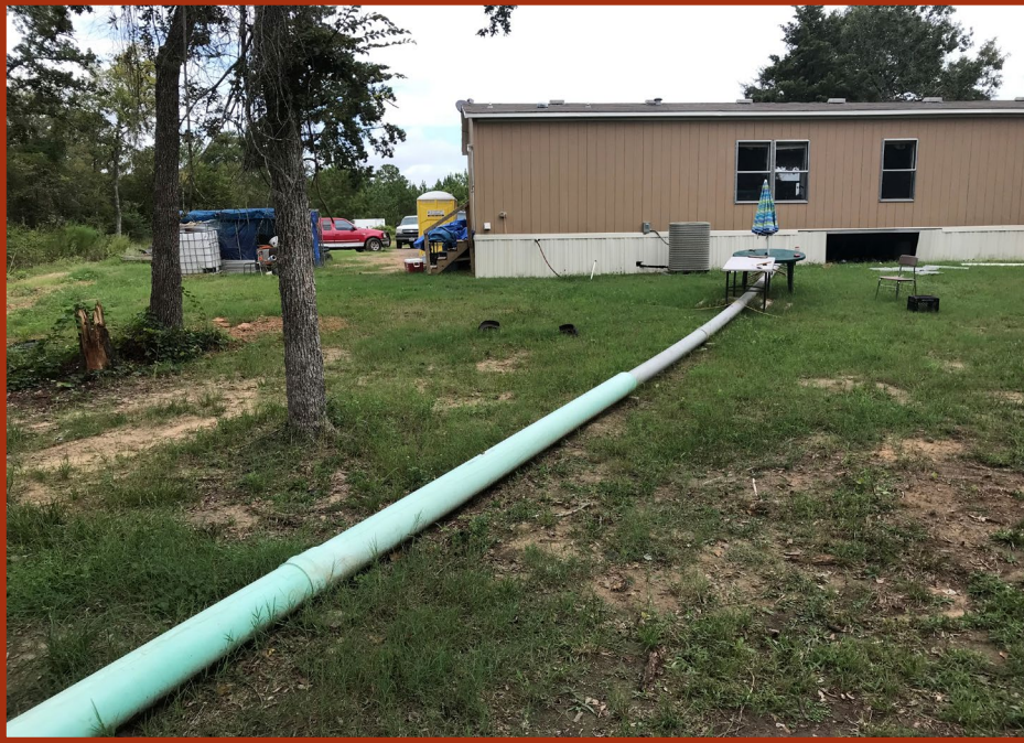
Pipe discharging to field
