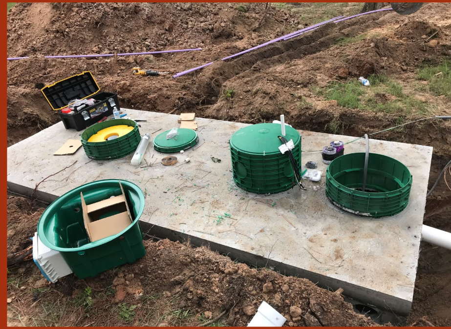
Installation of new aerobic system
